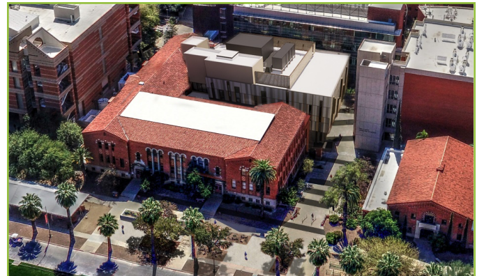
Chemistry Building Renovation
